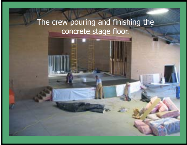
Wayne doing a bit of concrete finish work.
